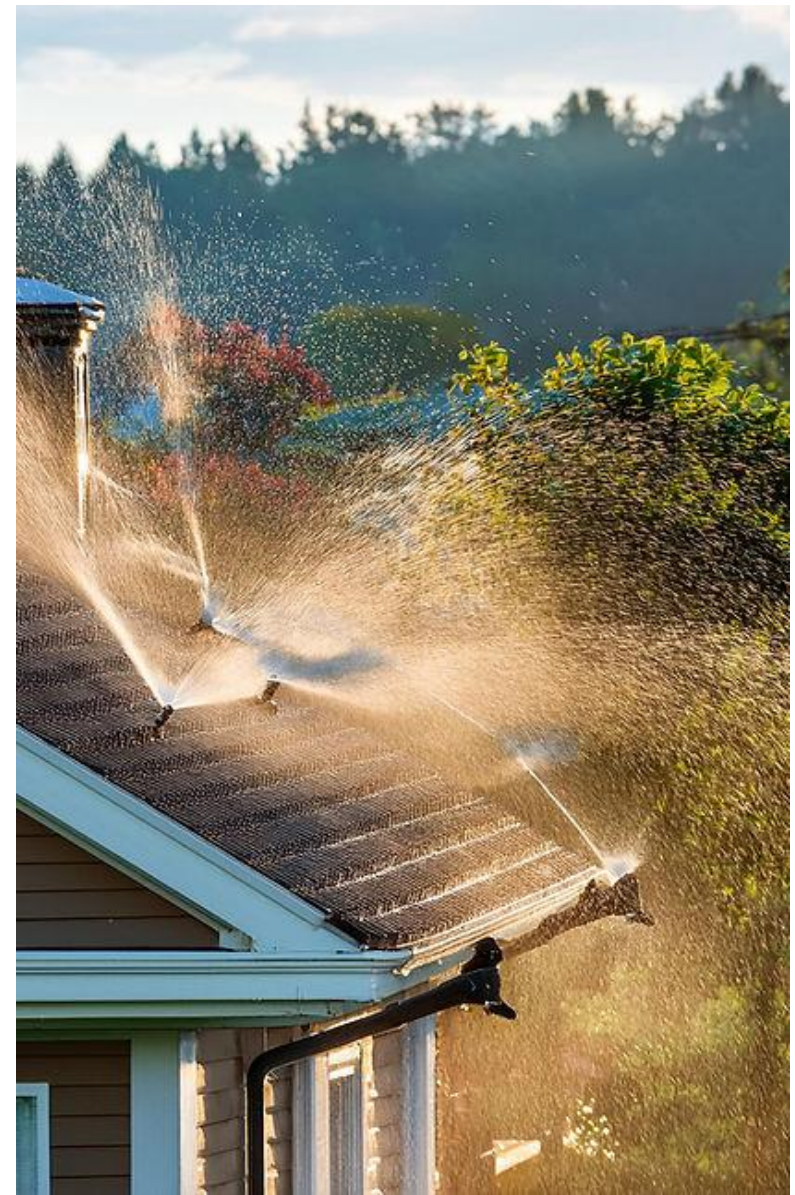
Photo Source: Wildfire Roof Sprinklers
